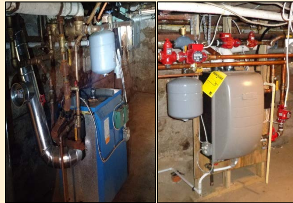
Before & After Boiler Replacement
